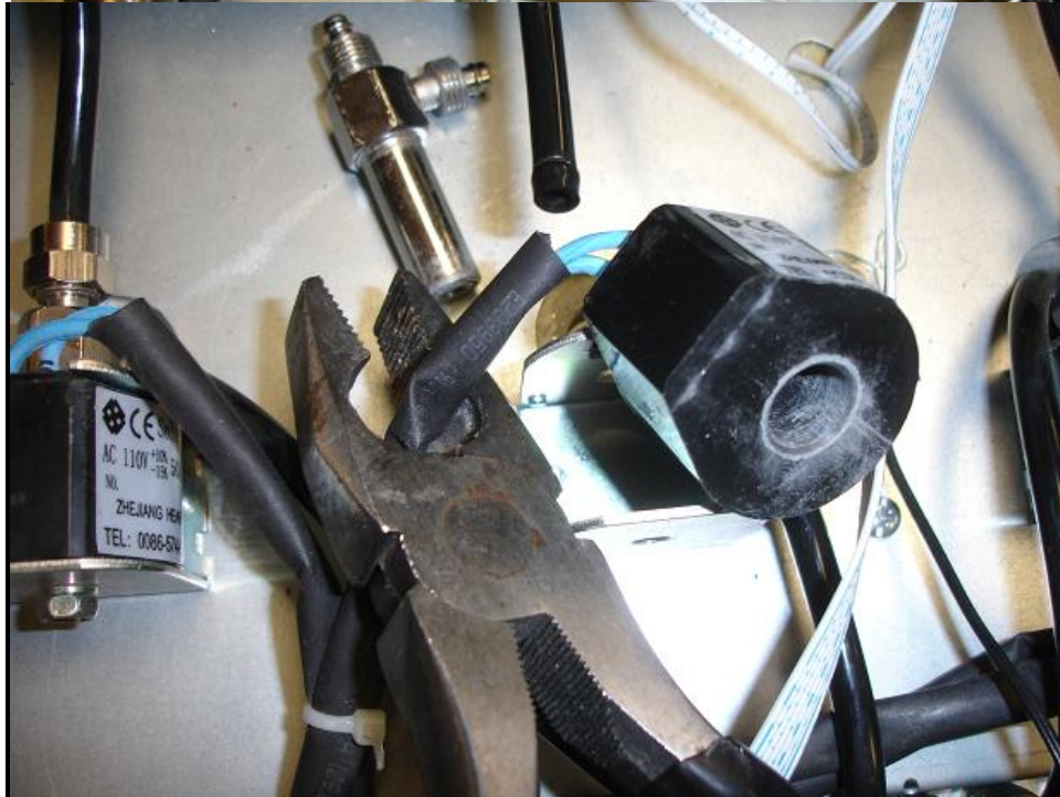
Cut the wires to replace the coil.
