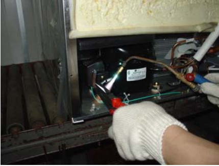
1-4-9. Replace it with a new process tube
