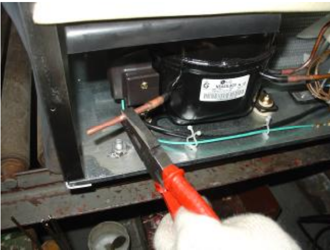
d. Weld the process tube
