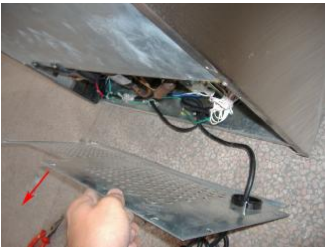
(4) If compressor is shaking when you touch it by hand, this shows compressor is working.
