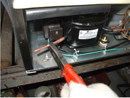
1-4-7-4、 Fix the process tube by welding.
