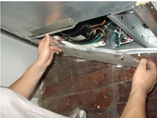
6-1-3、 Take off the screws of the control board cover (according to the picture)
