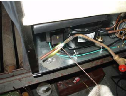
1-4-7-5、 Install the vacuumizing connector onto the process tube.
