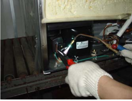
1-4-7-3、 Replace it with a new process tube
