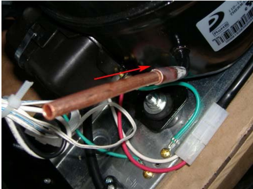
d. Fasten the new process tube with a welder.
