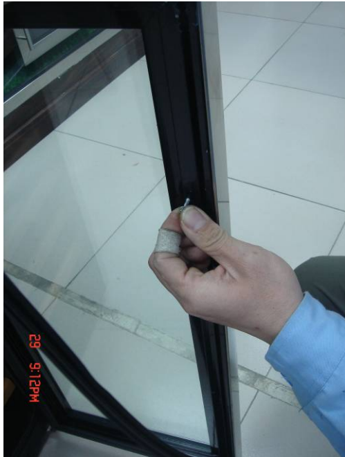
Step 3 Insert the screw
