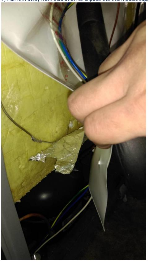
8) Pull the capillary tube out of its compartment, and reverse the process to install new thermostat.
