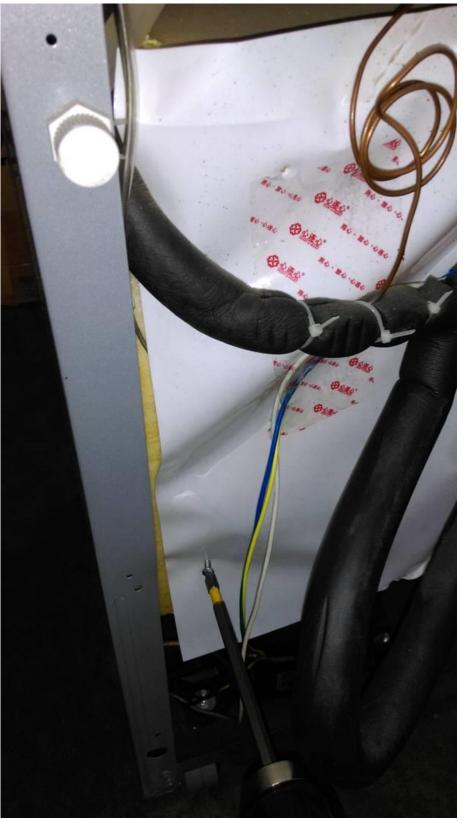
7) Pull film away from insulation to expose the thermostat capillary.
